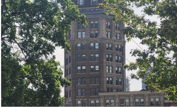
The Vancouver Sun Building
